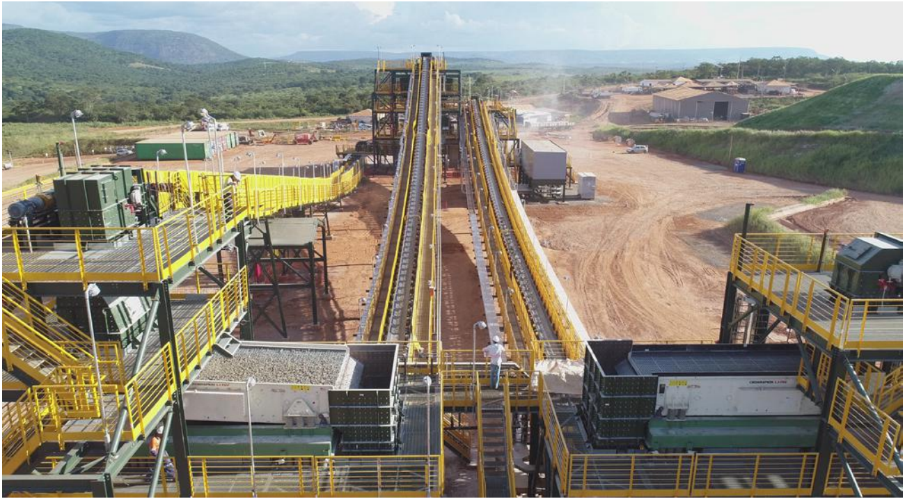
Sigma Lithium plant in the Lithium Valley
