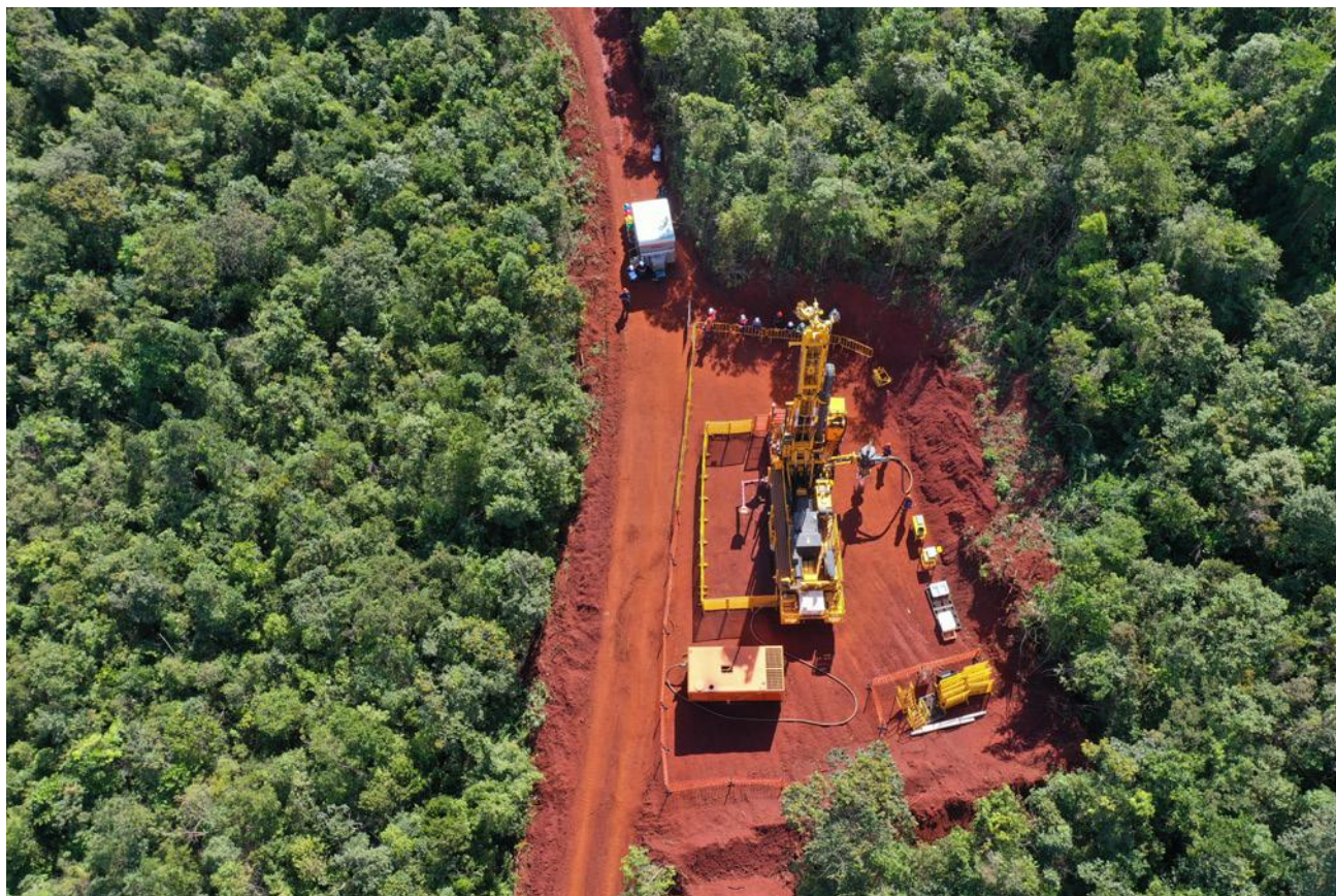
Geosol drilling operation
