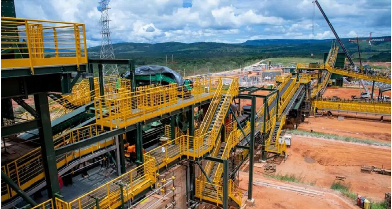
Sigma Lithium facility in Minas Gerais
