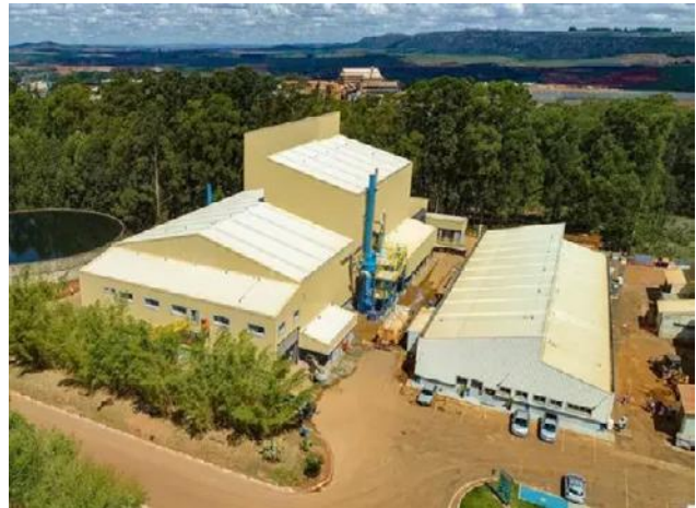
New CBMM plant at Araxá
