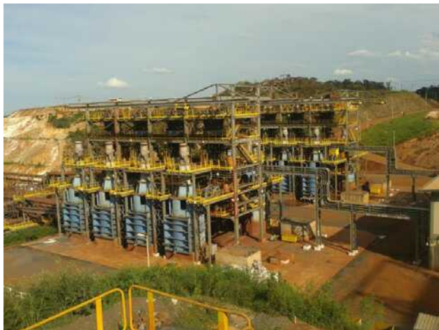
Grinding units at an Anglo American mine
