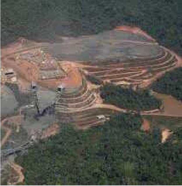
Vale's Salobo mine
